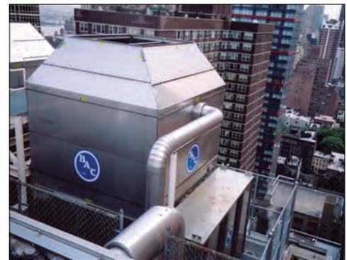
Unit with Intake and Discharge Sound Attenuation
