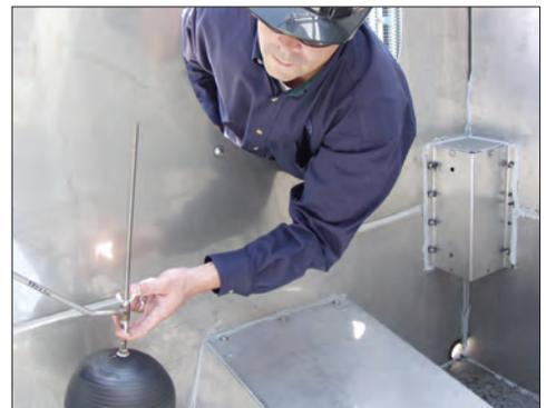
Standard Mechanical Water Level Control
