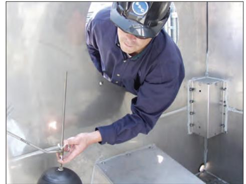
The Water Level Control is Easily Reached From the Access Door
